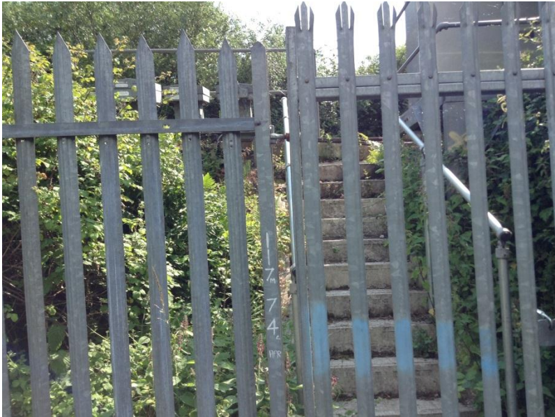
Figure 6: possible site access to Chittening station. A ramp would be required as well as the steps to access the platform.
