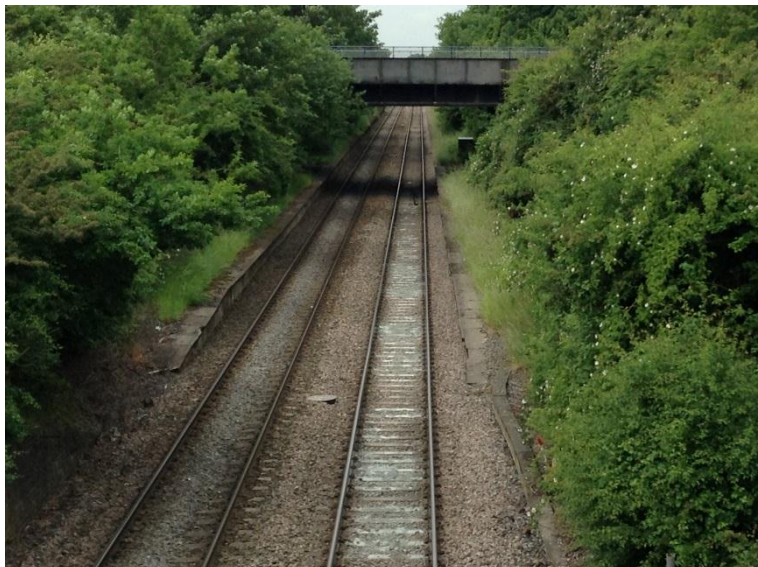
Figure 2.2 North Filton platforms from A38
